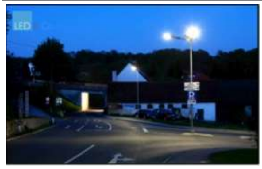
Before: 3 * 80 W High Pressure Sodium
