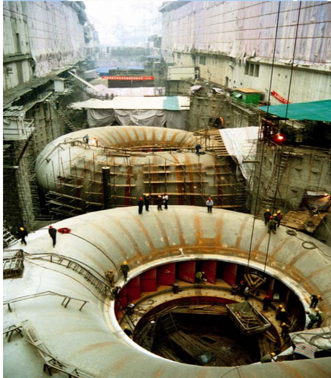
■ Spiral Case Installation
