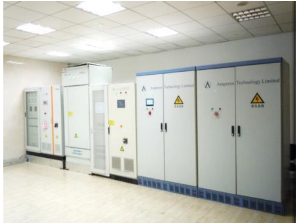
Capacity : 100 kW / 200 kWh Type: PV + Storage + Diesel
